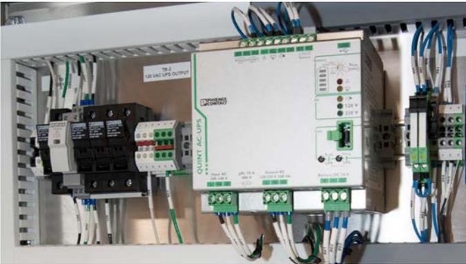
**Figure 3: Because the Class CC fuses are Class I, Division 2-approved, Xenon does not have to purge the panel.**
